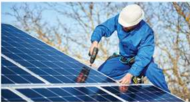
Solar Panel Installation
